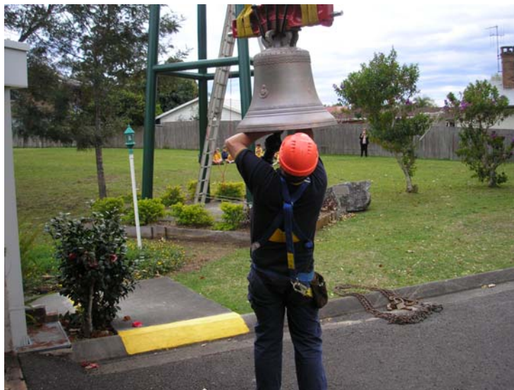
Securing the clapper upon installation
